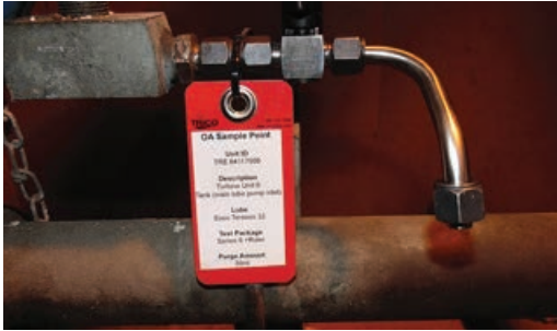
Figure 17: A properly labeled sampling point (Ref: Trico )
